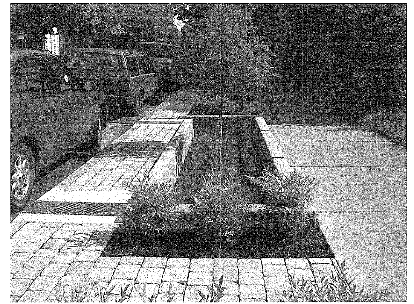
BASIN TYPE 'A' & PERMEABLE PAVERS
