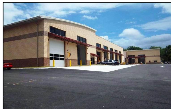
Renovation and expansion at the Newington DVS Facility in Mount Vernon District
