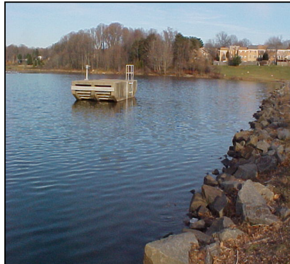
Photo of Lake Royal which is part of the County's extensive stormwater system.
