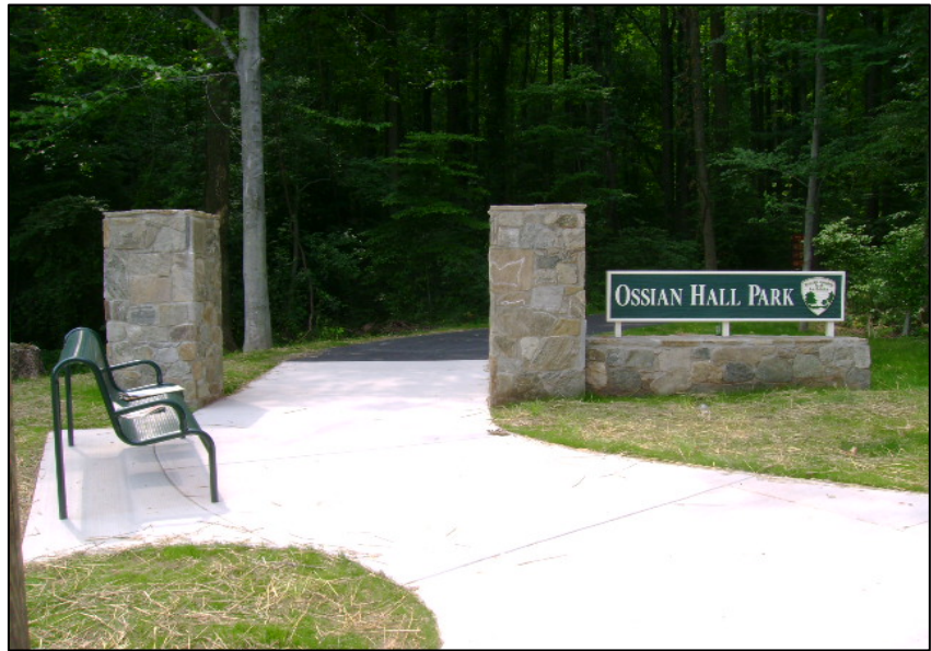
Ossian Hall Park – Phase I Improvements. The improvements were designed to provide better access and visibility into the park, located in Annandale, Virginia.
