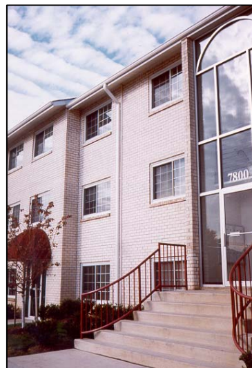
Murraygate Village apartments in Hybla Valley
