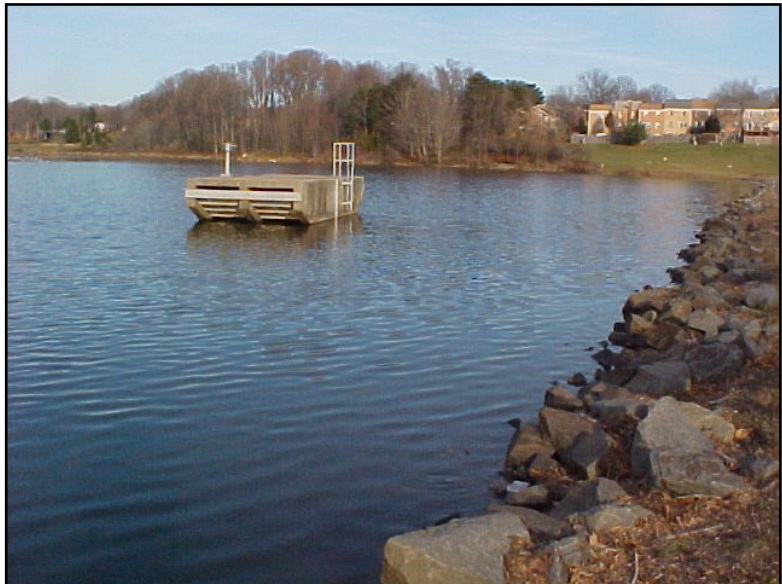
Photo of Lake Royal which is part of the County's extensive stormwater system that includes 1,800 miles of storm drainage conveyance systems, 45,000 stormwater drainage structures and approximately 1,200 publicly maintained stormwater management ponds.
